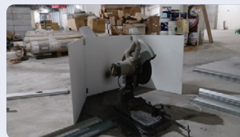
Use of fire-spark arrester to prevent sparks during grinding
