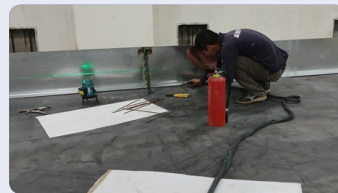
Face shield and fire extinguisher are in place for spot welding operation
